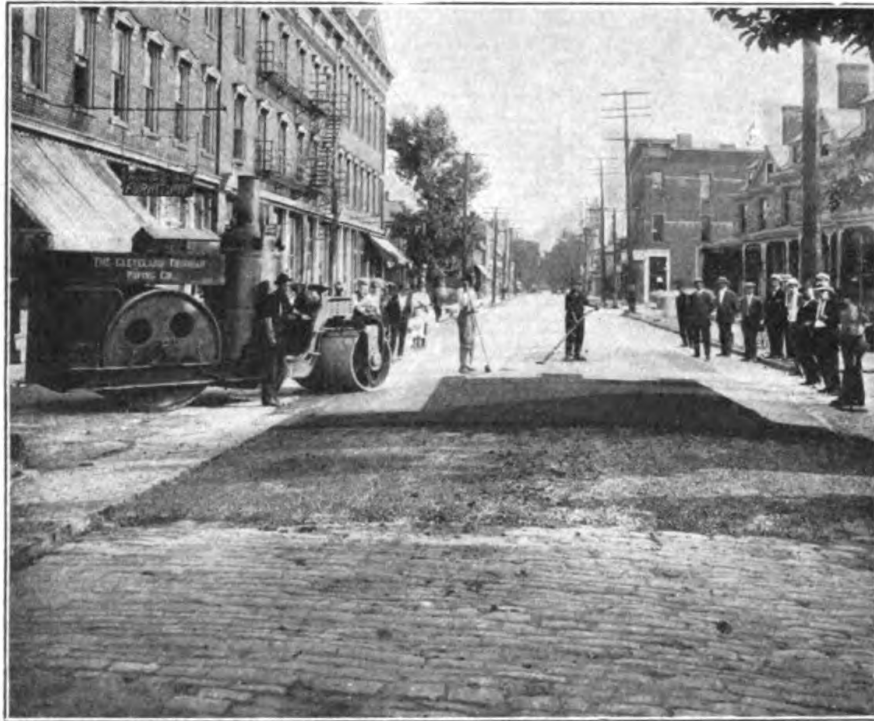
Resurfacing old granite block pavement with asphalt on Twentieth Street, north of Mt. Vernon Street, Columbus, O., 1915.
