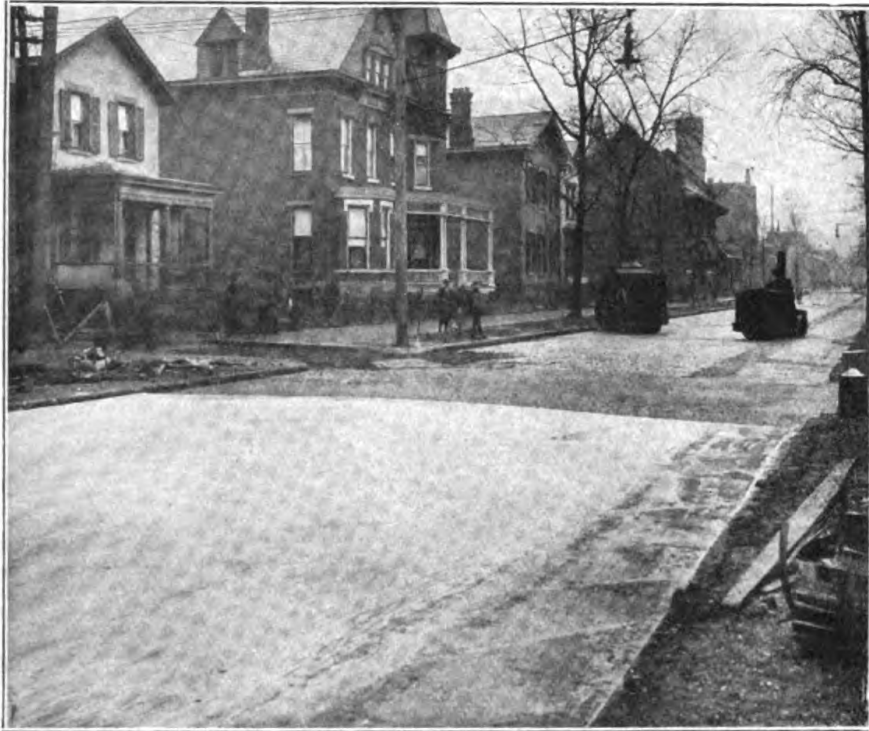
Sheet asphalt surfacing over old brick pavement on Sixth Street, Columbus, O., 1½-inch binder and 1½-inch top, 1912.
